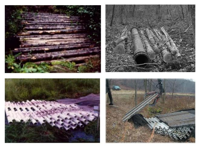
Figure 5-4 Examples of temporary log crossing structures with various types of fill-material, including slash only (top left) (Blinn, *et al.*, 1998); slash and pipe culvert (top right) (Aust, *et al.*, 2011), pipe bundle (bottom left) (Blinn, *et al.*, 1998) and pipe bundle with wooden panels overlain (bottom right) (Wisconsin DNR, n.d).
