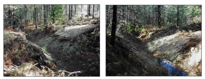
The situation was an ephemeral drainage line used during August, when the chance of measurable precipitation was minimal. The crossing was removed by September 1. There was no pipe or separator material used. Whole trees 250-600mm diameter breast height were used in the drainage channel. After the crossing was no longer needed, the material was removed with a heel-boom loader and processed at the landing. Standard erosion control measures where required.
