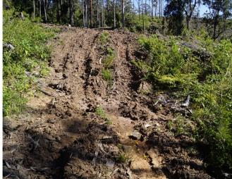
Causeway crossing showing disturbance associated with traffic during harvesting and site preparation for replanting. Soil in the drainage feature has been disturbed and could be mobilised during a significant rain event
