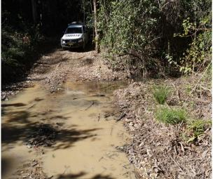
Causeway crossing in on-going use, with evidence of sediment generated following vehicle passage. Note that this is a road rather than temporary track crossing.
