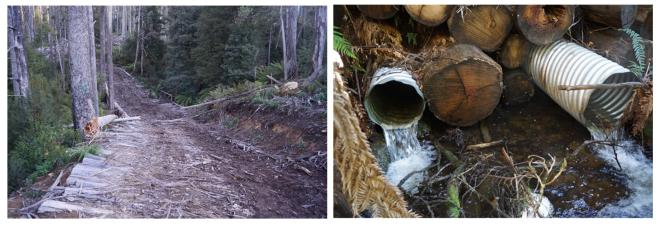
Figure 5-3. Temporary log crossing in use as a forwarding track across a permanent stream in tall, wet eucalypt forests in Victorian Central Highlands region. Source: Jacobs (2020).
